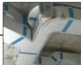
preinsulated aluminium air duct with self-cleaning and antimicrobial treatment
