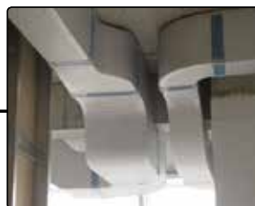
preinsulated aluminium air duct with antimicrobial treatment
